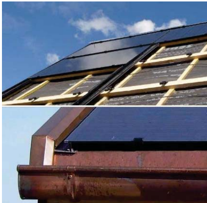
Slika 152: Ulaganje laminatnih panela, Samuel Summermatter, BE Netz AG
